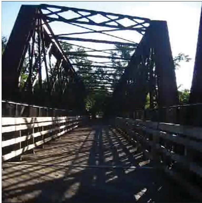
41 Still from bridge video.
